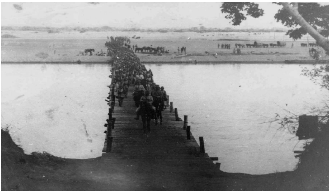
Trestle bridge over the River Rovuma built by the Portuguese forces in north Mozambique.
