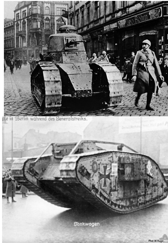
Figure 15 – The FT-17 weighted \frac{1}{4} of an Mk IV and had \frac{1}{4} of its crew, but in most combat situations could bring the same volume of fire to bear on a single target and was better armoured. It could also be moved around in truck.
